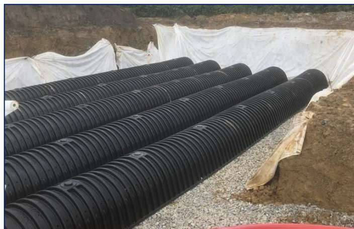
Figure 3.8 – Typical Poly-Tunnel Installation Arrangement
